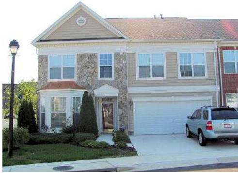
Stone veneer on front elevation
