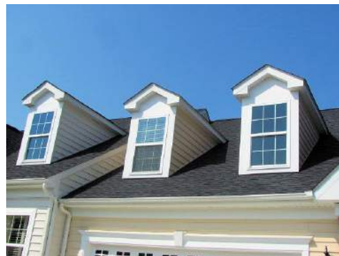
Composite trim at soffits, rake and dormers
