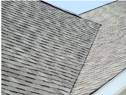
Asphalt shingle roofing
