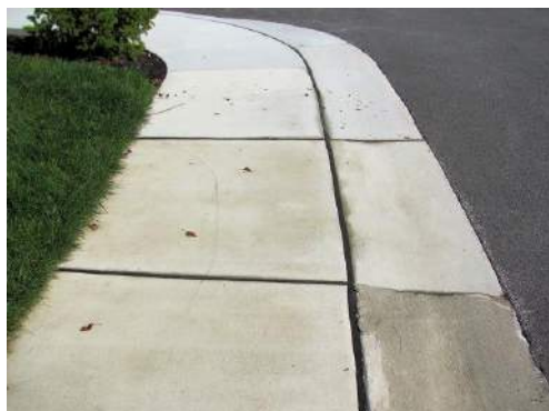
Typical sidewalk and gutter. Note: section of both have been replaced
