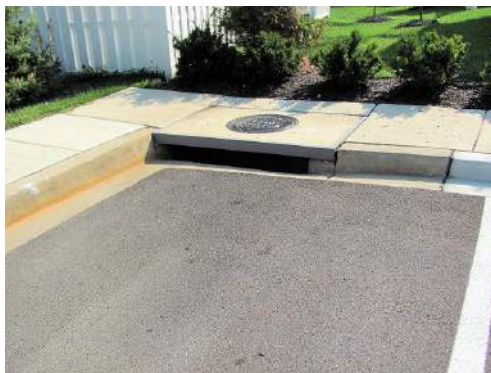
Typical street drainage unit
