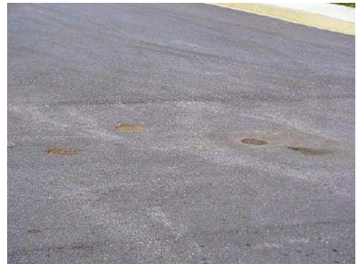
Asphalt pavement with water control boxes
