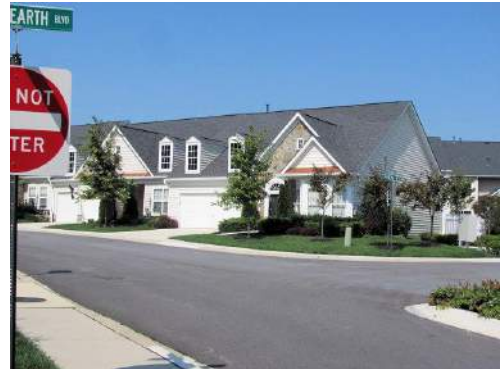
View of one story roofs and dormers
