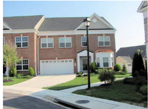
Brick veneer on front elevation
