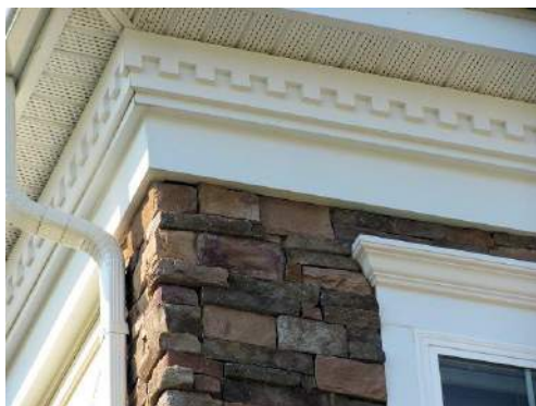
Composite frieze and dentil molding at soffit area
