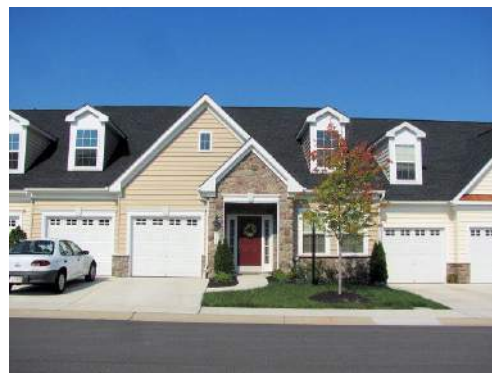
Vinyl siding at front elevation
