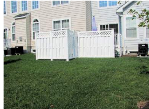
Typical vinyl fence at mid-unit of building
