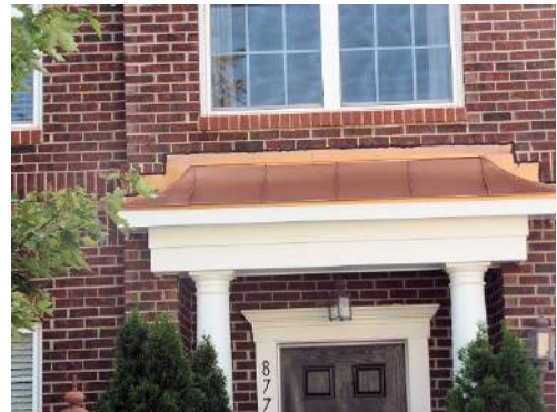
Metal roofing above small building entrance roof
