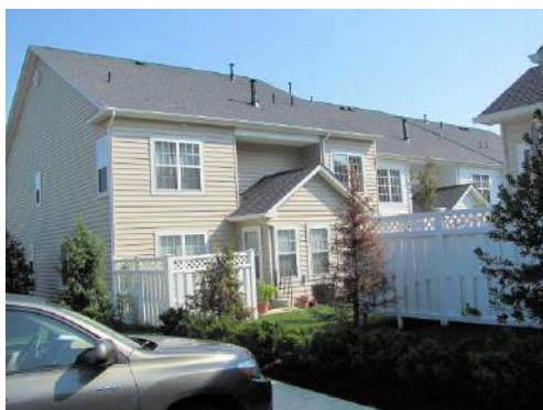
Vinyl siding at rear and side elevation
